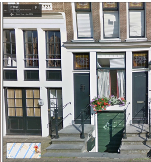
Closed window at the canal
