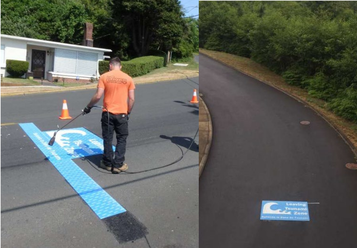
Figure 3. Tsunami blue line signage in (a) Newport, OR (courtesy of Mike Eastman) and (b) Seaside, OR (courtesy of Anne McBride).
